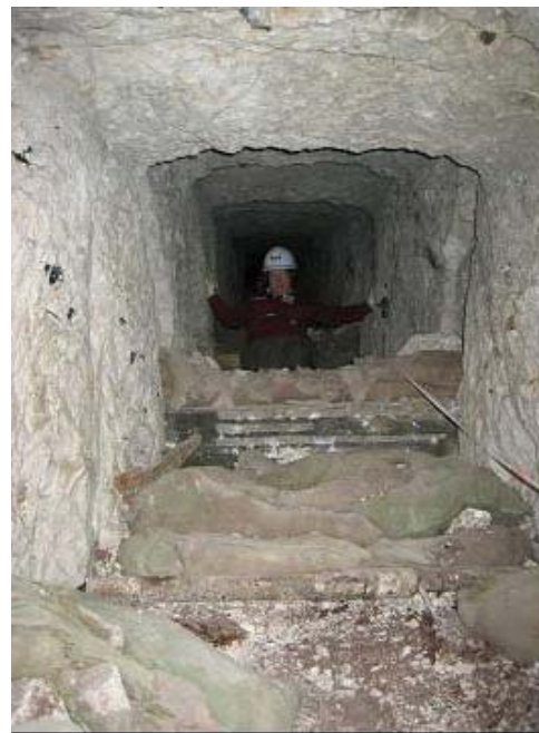
Figure 2 and 3: Tunnels remaining from WWI at the Vimy Ridge Memorial Site. The photos show the condition of the chalk near the ground surface (top), and at approximately 20m depth (below). Access to these tunnels was only recently re-established.
