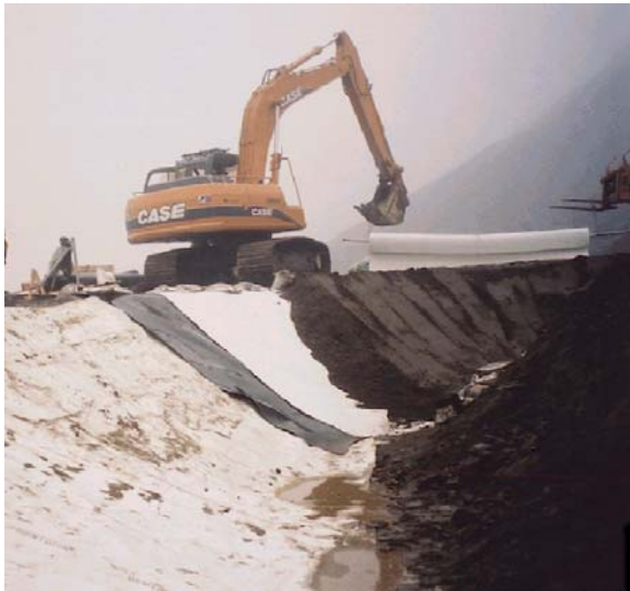
Installation of barrier system in 2001
