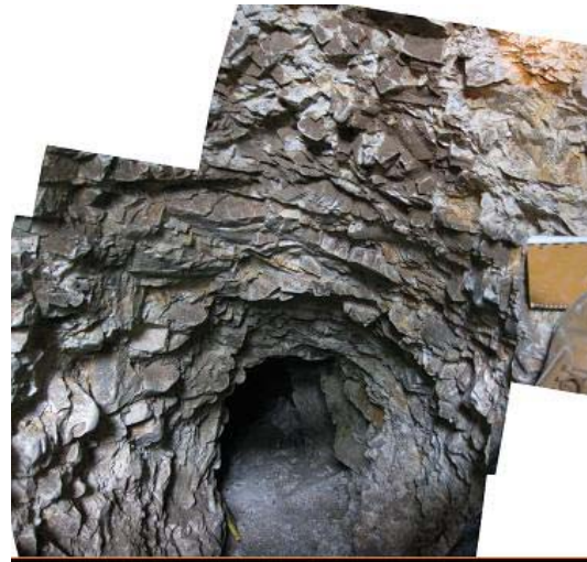
Figure 2 and 3: Tunnels remaining from WWI at the Vimy Ridge Memorial Site. The photos show the condition of the chalk near the ground surface (top), and at approximately 20m depth (below). Access to these tunnels was only recently re-established.
