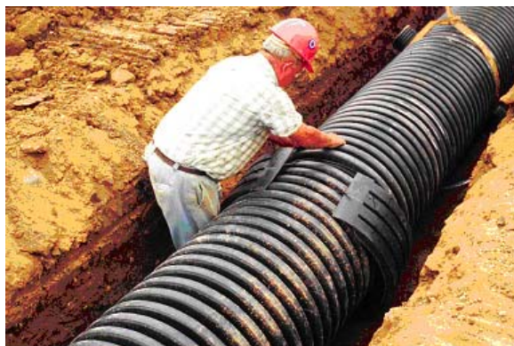
Profiled HDPE pipe being installed near Chatham, Ontario
