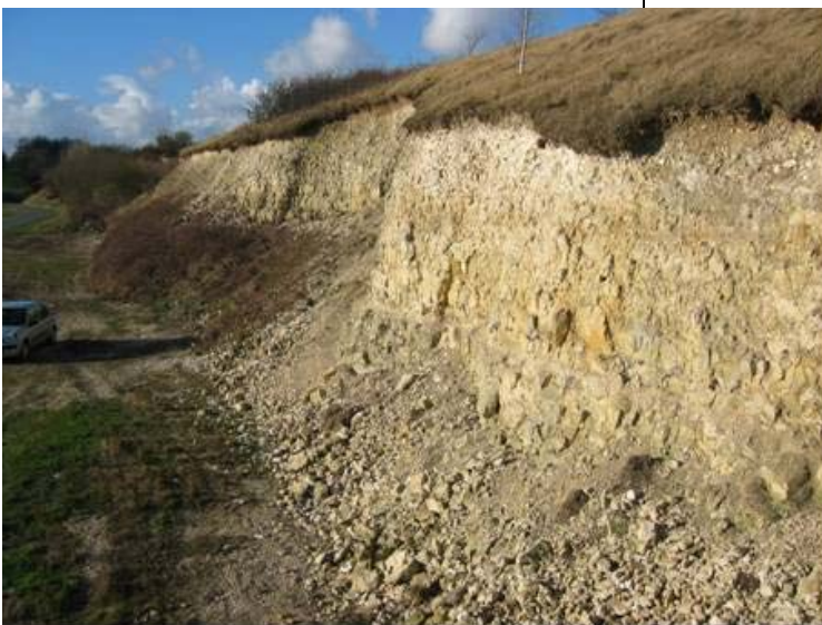
Figure 5: Condition of the rockmass exposed in a quarry, near Beaumont Hamel Memorial Site.
