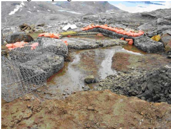
Funnel and Gate Barrier under Construction, 2004 Field Season
