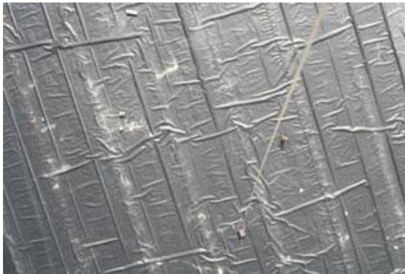
Figure 3 Air photo of geomembrane installation. 1.5 mm smooth HDPE; Camera
