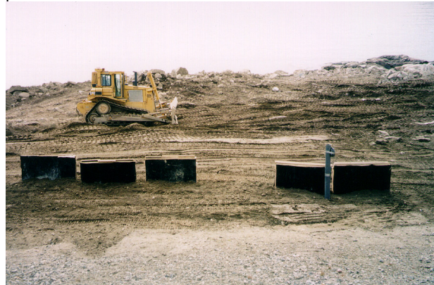
Figure 3: The frames supporting f-HDPE GM coupons during installation in 2001
