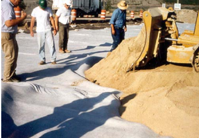
Figure 13 Photo showing wrinkles (Photo courtesy of R. Thiel).
