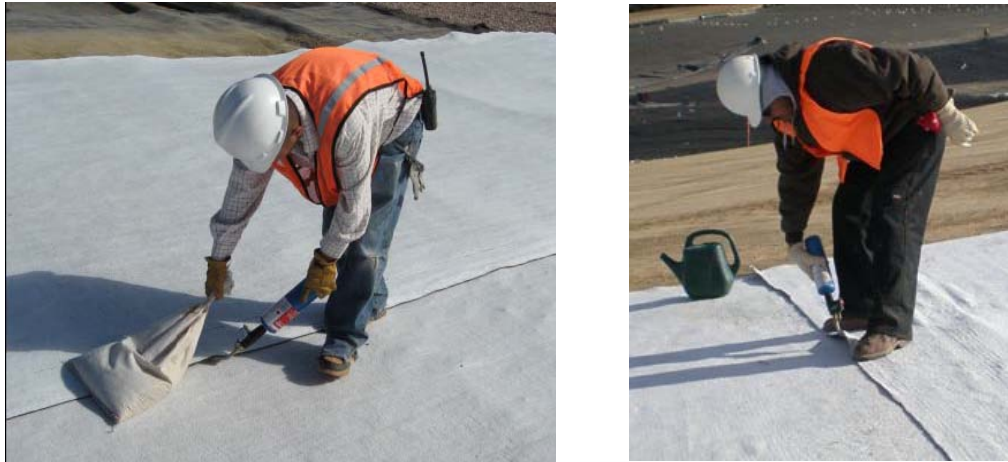
Figure 6. Installer heat-tacking GCL edge seam with a 0.15 m overlap.
