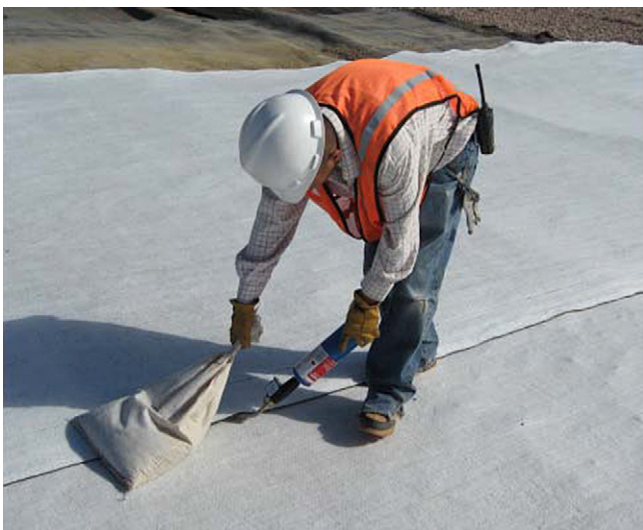
Fig. 1. Heat-tacking GCL panels with a 150 mm overlap to form a seam.
