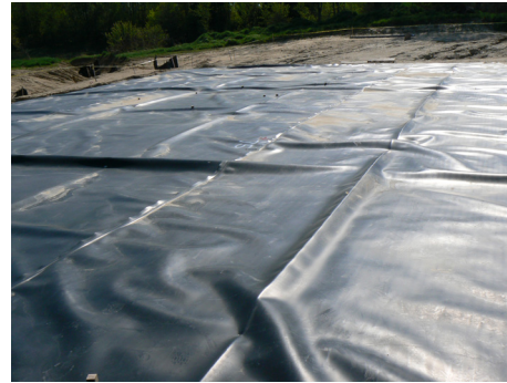
Figure 2. Interconnected wrinkles in a GM; midmorning when ambient temperature is 17°C (same location as shown in Figure 1)
