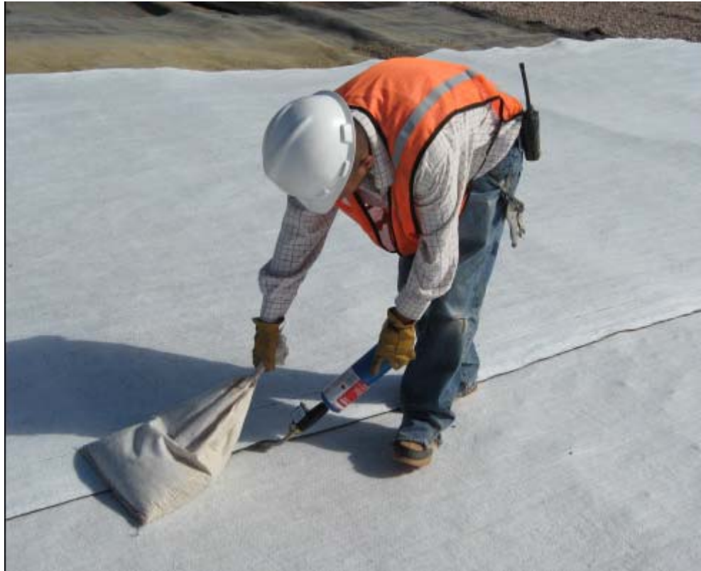
Figure 1. Installer heat-tacking GCL edge seam with a 150 mm overlap.
