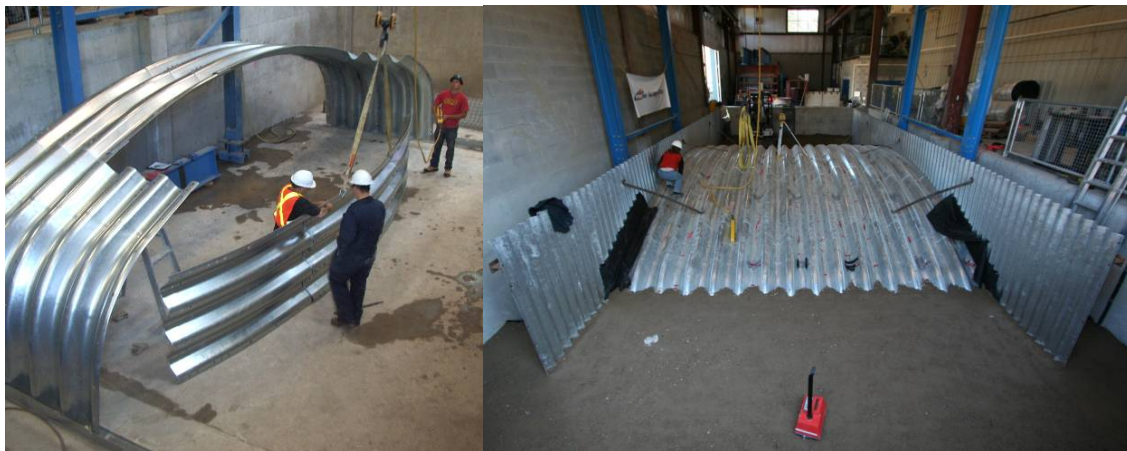
Figure 2. Culvert erection and backfilling.
