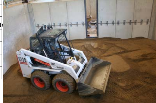
b. Placement of foundation soil.
