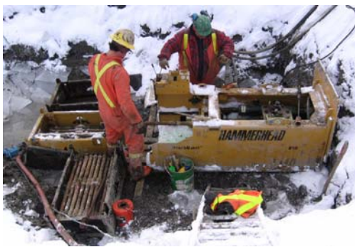
a. Pipe bursting equipment in use in Ottawa, Ontario
