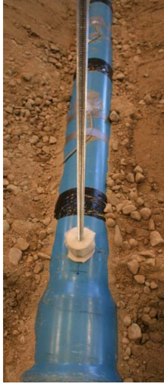
d. Rod to monitor pipe uplift
