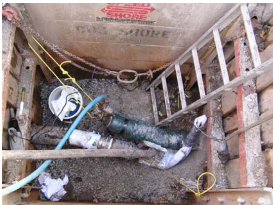
Figure 4. Liner inflation and curing using hot water
