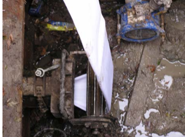
Figure 3. Resin impregnated liner pulled into place.
